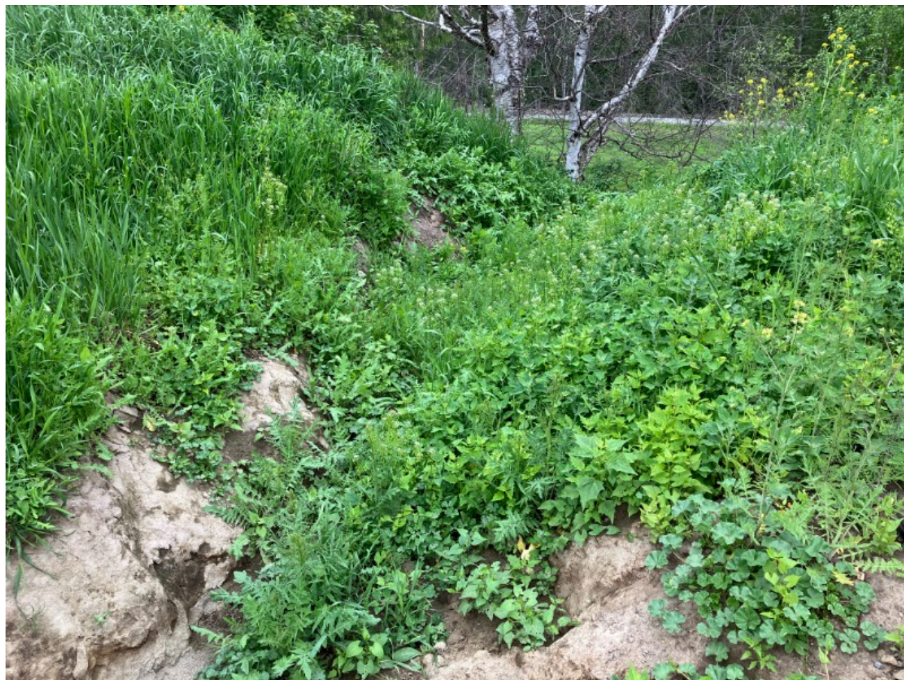
Photo 4. Westward bank adjacent to the confined livestock areas, where the drainage pipe enables contaminated runoff to escape.
