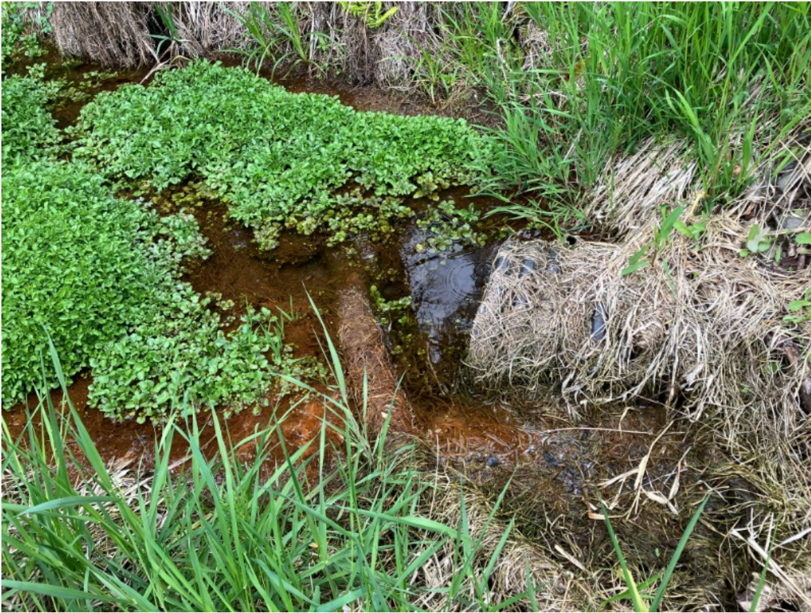
Photo 5. Ditch with culvert where the contaminated runoff crosses the neighbouring property boundary.
